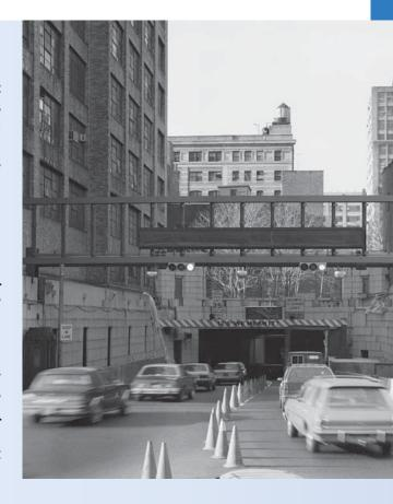
Ventilating the 1.6 mile tunnel posed a significant engineering challenge. A two-duct ventilation system was developed that, with its eighty-four immense fans and four ventilation buildings, can completely change the tunnel air every 90 seconds. Tests at the time showed that air quality in the tunnel was cleaner than in Midtown Manhattan.
