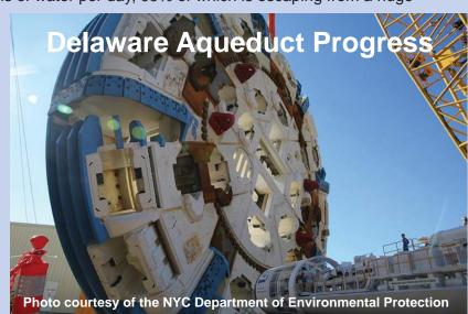
the TBM's 21.6-ft. cutter head will begin boring through about 50 feet of rock per day, all while pumping 2,500 gallons of water per minute, installing a concrete lining, and conveying pulverized rock to underground rail cars, for the next twenty months. Finally, the tunnel will be reinforced with steel pipes and a second layer of concrete. A 6-month shutdown is scheduled for October 2022, at which time the bypass will be connected to the Aqueduct.
