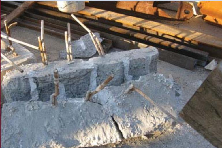
Chemical bursting is accomplished by pouring a slurry of expansive grout into boreholes drilled into the concrete in a precise pattern. The grout expands for up to a week as it dries, creating cracks within 12-24 hours and silently breaking the concrete into manageable pieces for easy removal by hand or crane. The process is safe, quiet, vibration-free, and produces little to no dust.
