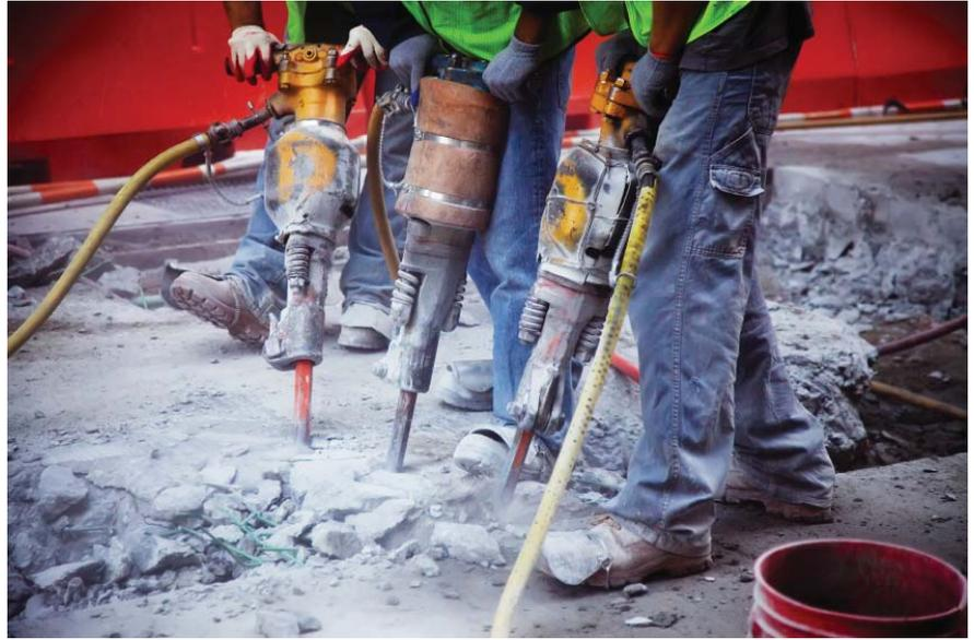
to change position and reroute compressed air beneath the piston, forcing the piston backward upward and releasing pressure from the ground. This repeating cycle produces up to 1,500 powerful blows per minute.
