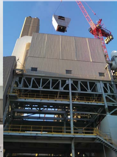
The lower half a 26,000 lb. front transition wall is carefully detached from the structure.
