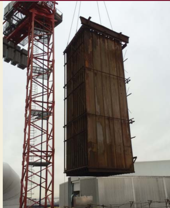
One of the facility's nine 30,000 lb. humida frame sections is lifted from inside the unit following removal of the roof.
