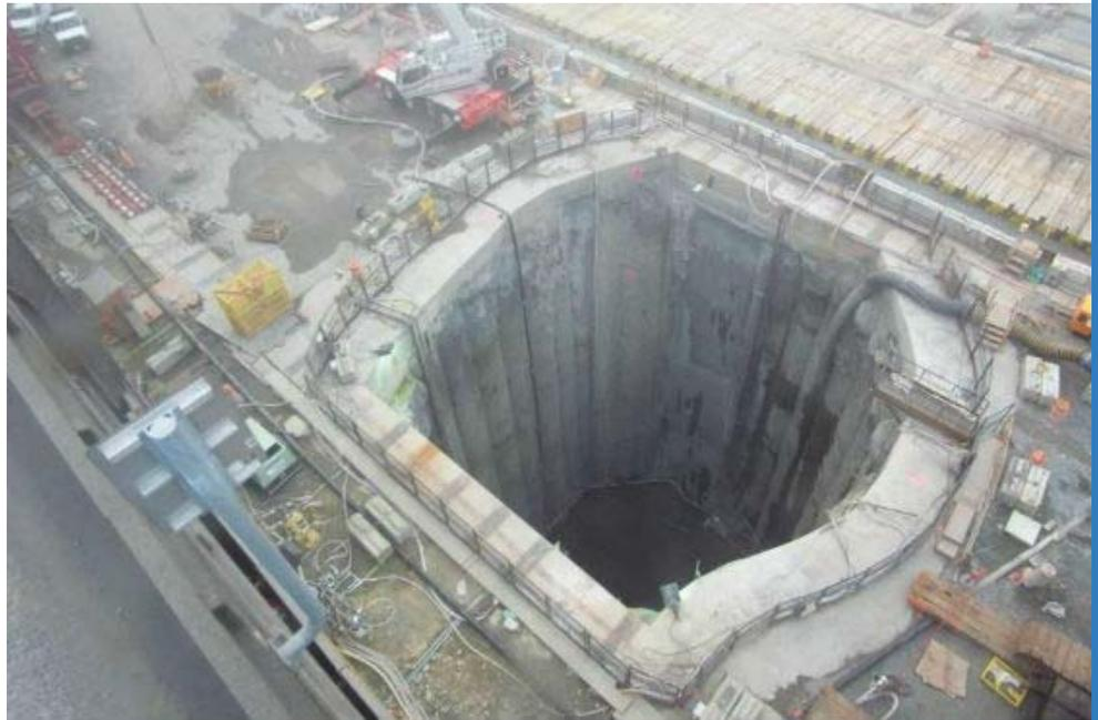
Once the front of the TBM is secured on the cradle, workers will detach the 57-foot diameter, 2,000 ton cutter head. A modular lift tower (MLT) will be moved over the pit to hoist the massive assembly to the surface, rotate it 90 degrees to the horizontal, and set it on the ground for disassembly and repair. Bertha's cutter head will receive a new bearing assembly, extended agitator blades, widened mouths to process more material, and
