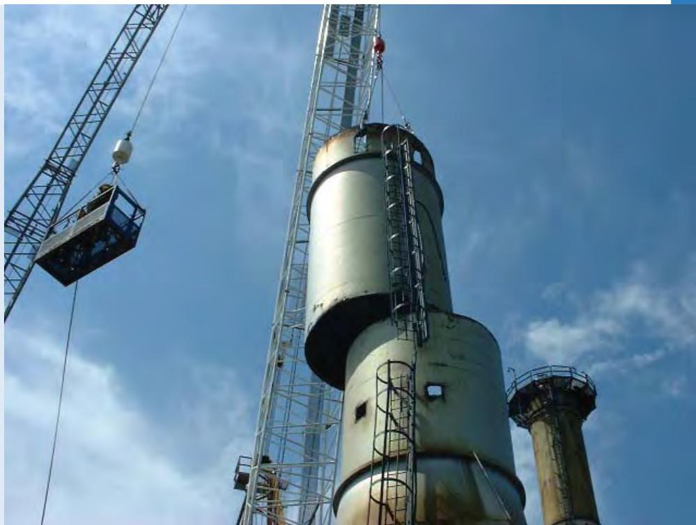
basket nearly 350 feet in the air to allow crew members to perform rigging and dismantling of the stack and breeching. **The project was complicated by the close proximity of live power lines, cooling towers, and the new powerhouse, which was required to remain online for the duration of the project.**
