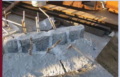
Chemical bursting is accomplished by pouring a slurry of expansive grout into boreholes drilled into the concrete in a precise pattern. The grout expands for up to a week as it dries, creating cracks within 12-24 hours and silently breaking the concrete into manageable pieces for easy removal by hand or crane. The process is safe, quiet, vibration-free, and produces little to no dust.
