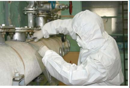
into the air. Materials that, if installed before 1981, should be presumed to contain asbestos include: spray-on fire proofing and insulation, insulation for pipes and boilers, wall and ceiling insulation, ceiling tiles, floor tiles, putties, caulks, cements, cement pipes, roofing and siding shingles, wall and ceiling texture, joint compound, and plasters. Almost all mechanical rooms constructed prior to 1981 will contain asbestos.
