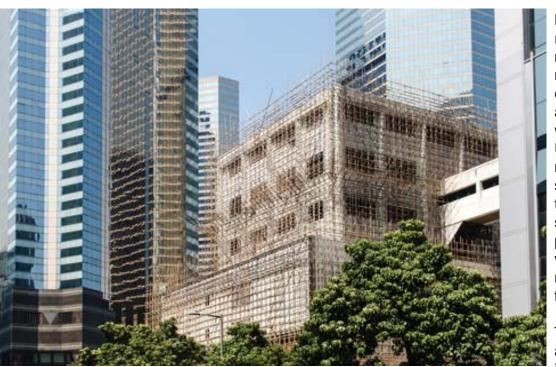
Bamboo is sturdy, lightweight, recyclable. and renewable. making it an ideal scaffolding material. Bamboo scaffolds are erected up to a thousand feet above the ground by skilled workers known as taap pang. Using very little safety equipment, the taap pang erect the spidery structures from twenty-three foot bamboo poles secured with plastic ties. Completed scaffolds are enveloped colorful nylon fabric, making the buildings looks like festively-wrapped gifts.
