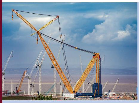
The ring crane is a type of luffing jib heavy-lift crane with a broad, round track at its base that allows the slewing while carrying extremely heavy loads. Ring cranes, which are relatively uncommon, have long reach and a small footprint and can lift as much as 5,000 tons. They are typically used in the construction of refineries, oil and gas, mining, offshore platforms, and nuclear power plants.
