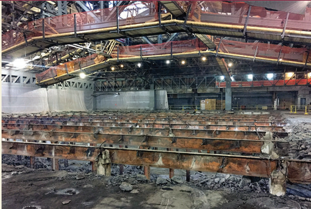
Exposed steel beams where the concrete floor has been removed. A second layer of concrete sits ready for demolition.
