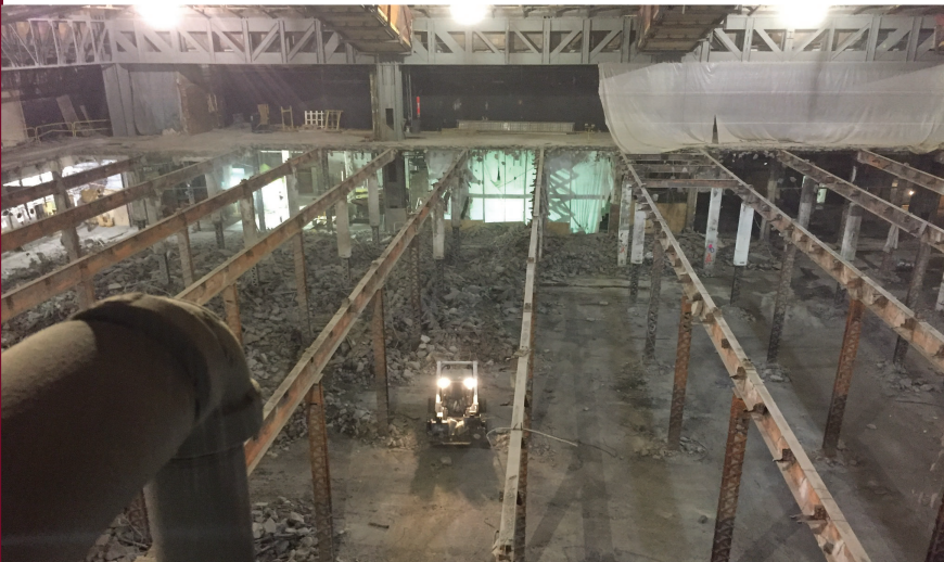
A skid steer loader removes concrete debris from the future main concourse.
